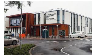
Boyle Primary Care Centre
